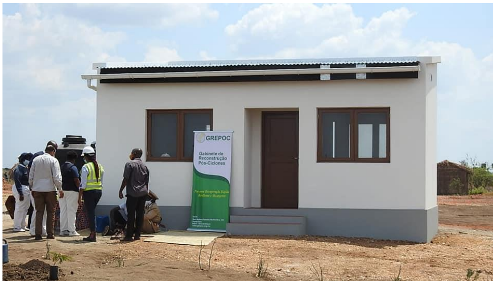
Figure 10 Residences constructed by GREPOC in safe zones identified using geospatial information
