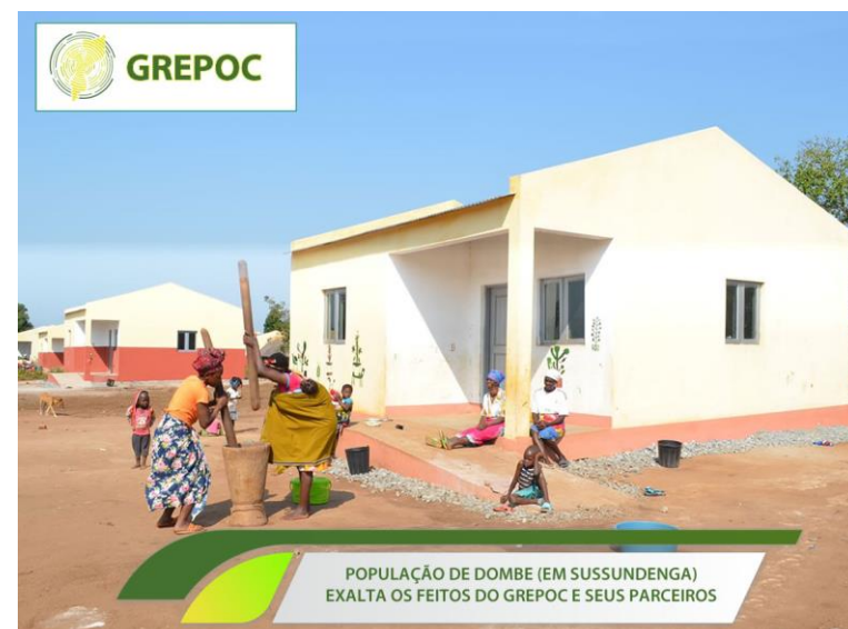
Figure 11 Residences constructed by GREPOC in safe zones identified using geospatial information
