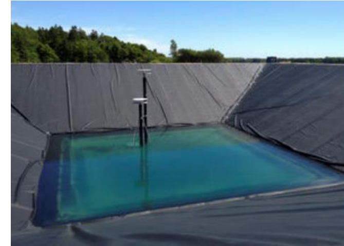
Pit Thermal Energy Storage (PTES)
