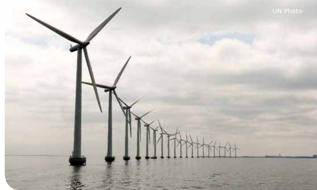
Middelgrunden offshore wind farm in Denmark
