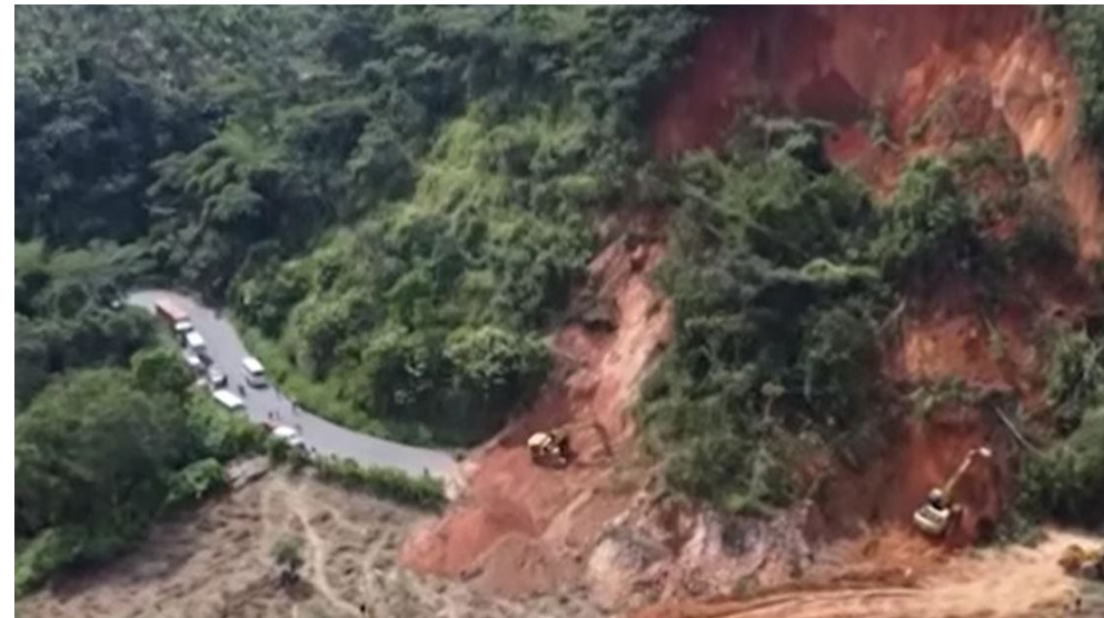
Double landslide on the Dschang road, 2024, killed at least 25 people.
