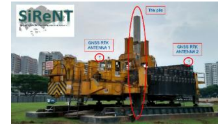
GNSS Assisted Piling System
