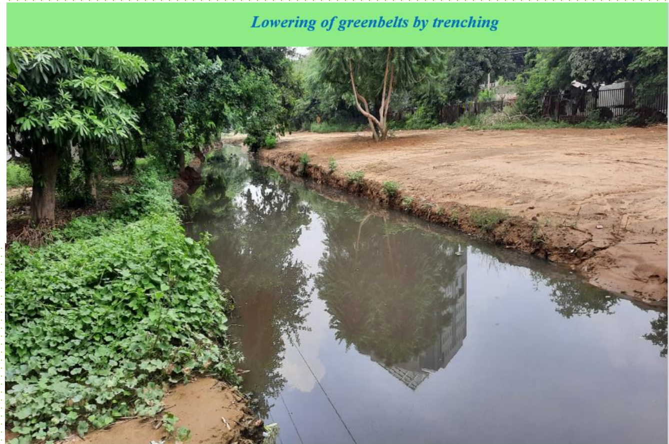
Lowering of greenbelts by trenching to hold water Sector 27, near Max hospital
