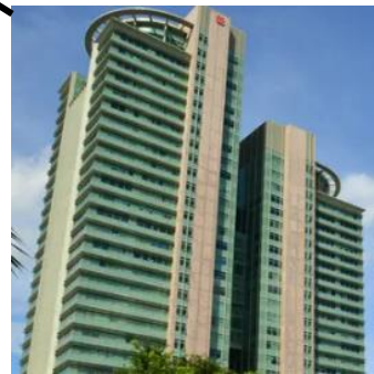
HDB Hub (Building)
