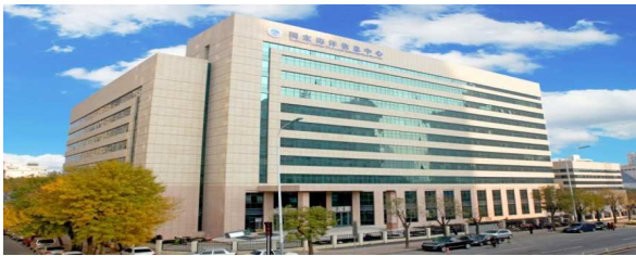
New look after energy-saving reconstruction in September 2016
