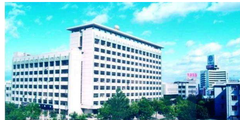
Office building in April 1989
