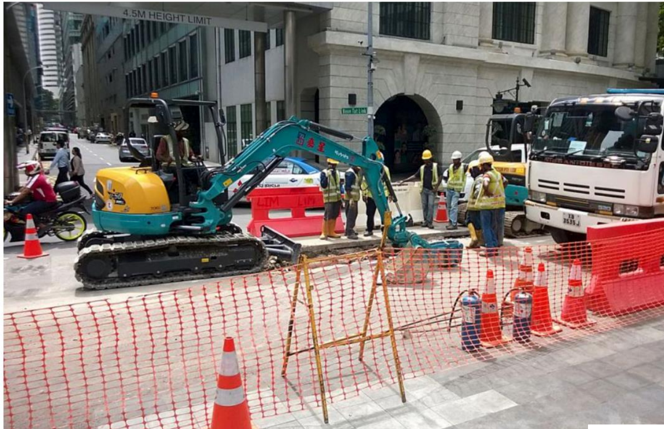
Boon Tat Street was cordoned off because of the gas leak, but gas supply to the area was not affected. Photo: Robin Choo
