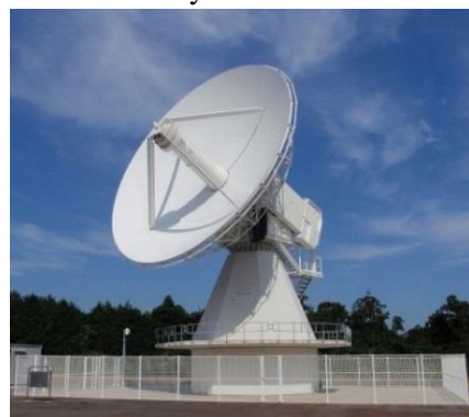
Ishioka VLBI observation facility
